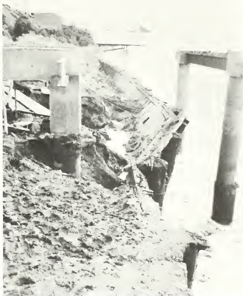
FIGURE 128.—View from the landward side, showing extreme damage to the seawall at Malibu Beach, Calif., produced by the wind-reinforced erosion, and undercutting of the seawall from the rear caused by these augmented high tides.
